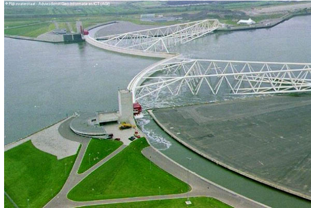
Figure 0.5: The Maeslantkering fully closed along the Nieuwe Waterweg. (Source Rijkswaterstaat)
